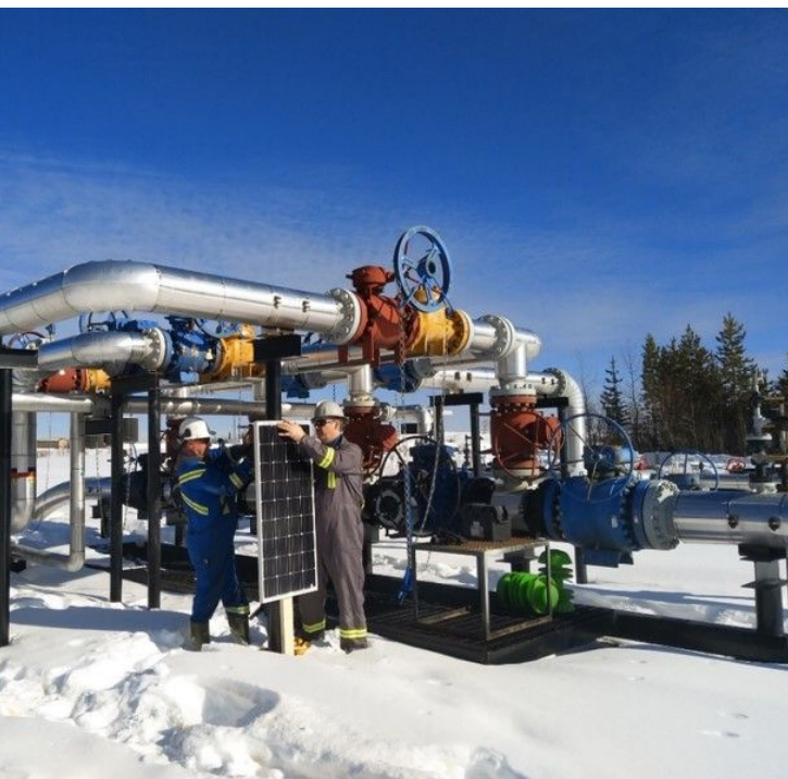
Installing Symroc Sensor on an Oil and Gas Facility
